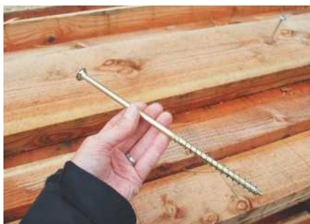
The mammoth screws used for fixing the Machinery Store's larch panels
